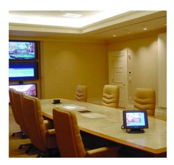
Controlling audio/video and lighting is a Crestron system comprising twenty CP2E controllers. Seventy-five Crestron lsys TPS-2000L touchpanels are used throughout the meeting rooms for simple selection of discrete audio channels. Nine Crestron MT-500C MiniTouch handhelds control the corporate suites. Crestron CNX-DVP4 digital video processors interface with Crestron TPS-5000 15" touchpanels for display of four real-time video/computer windows and two high-resolution document cameras.
