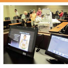
Crestron DigitalMedia was installed to handle high definition signal routing, switching and long distance distribution of all analog and uncompressed HD digital signals throughout the facility. CresFiber® supplied the long distance AV distribution, transmitting all signals up to 1000 feet. The distribution of DigitalMedia enables live demonstrations in one location to be viewed by faculty and peers in another classroom on another floor.
